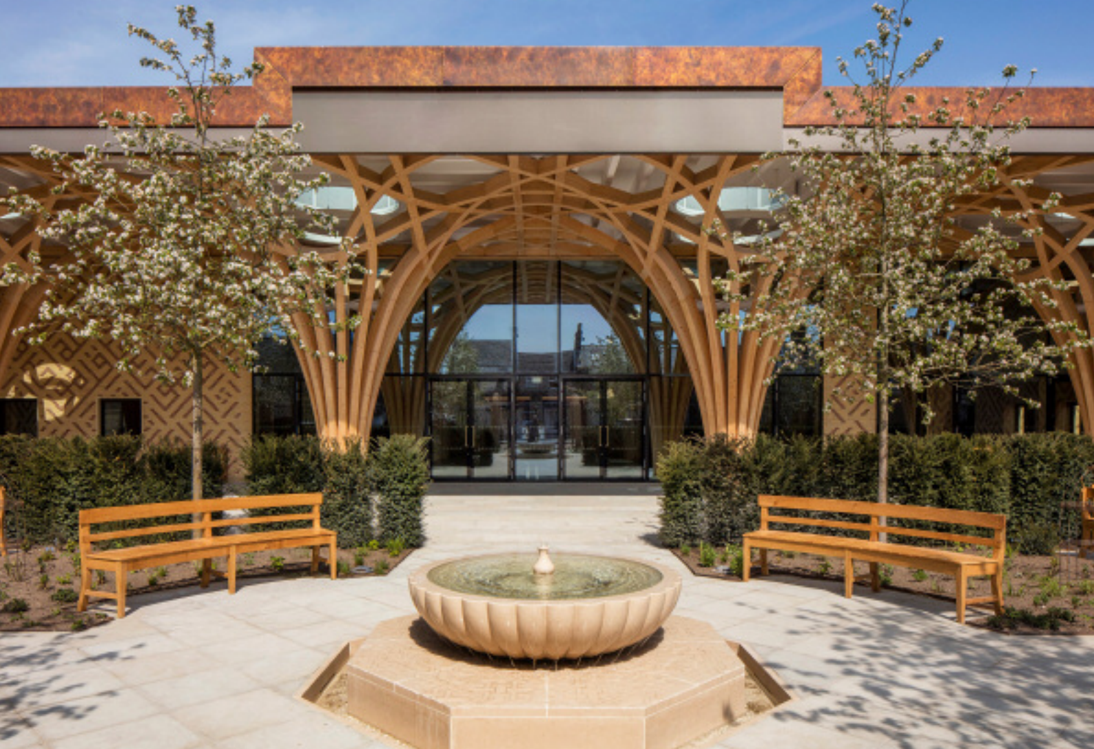
The new Cambridge Central Mosque; the Islamic gardens, the font and the front portico. The 'breath of compassion' geometry seen on the entrance pillars continues in the interior. Photograph: Morley von Sternberg
